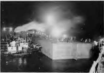
WHILE QUEEN JULIANA watched, seven powerful tugs pushed a huge caisson into place at Ouwertrek. It was a joyous moment for all Holland. The date was Nov. 6, and it marked the closing of the last and biggest gap in the many breaks the dykes suffered. RAO YUSTA DI BRINA JULIANA, siete potente remolcador e hala un arcon grandi pausa na su lugar na Ouwertrek. Tabata un momento alegre pa Holanda. E fecha tabata Nov. 6 y ta marca cerramiento di ultimo — y mas grandi — buraco di e cantidad innumerable cu tabatin den e dijknan.
